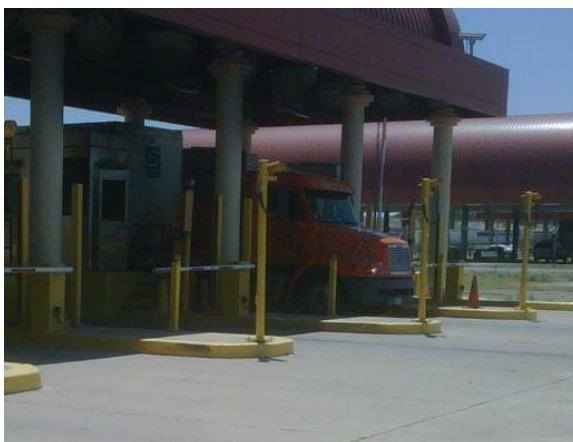
IZDVAS Solution Deployed At The International Bridges System In Texas
